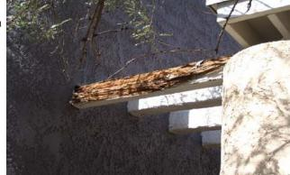
Dry rot affecting roofing support structure at pool area ramada roof - The stucco-wrapped asthetic beams are a design deficiency as they serve no structural purpose, and are compromising the structural soundness of the attached roofing structure. As seen in this photo, the beams are trapping water at the joints, which is causing dry rot not only in the beam, but also in the roofing support beams of the ramada roof structure.
